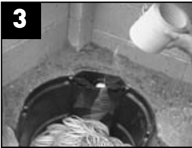
3 Hold filter media, pull from the bottom center of the roll. Media will self dispense to fill filter chamber.
