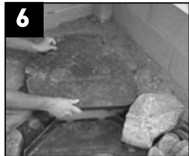
6 Put lid into place, secure with bolts provided. Start pump and allow filter to fill with water.
