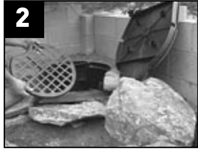
2 Lower media grate into position.
