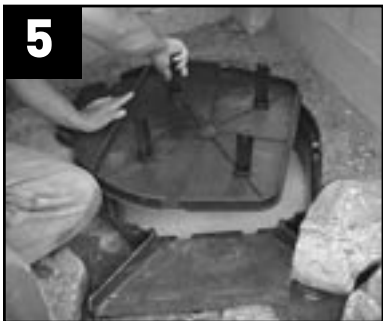
5 Insert media stabilizers into underside of lid.
