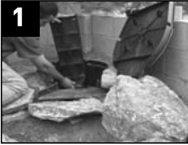
1 Slide baffle down grooves inside filter.
